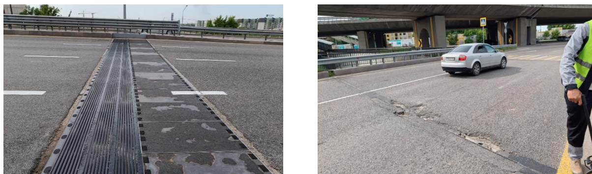
Figure 2. Transport interchange and exits on the Northern Ring Highway, near Salem Shopping Centre, city Almaty [photos taken by the author Bondar I.S.]
