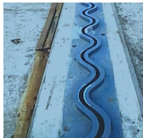
Figure 10. Photographs of the OP-DSH-K2-in wave-shaped border [the drawings are taken from the website https://k2-engineering.ru/produksiya/deformatsionnye-shvy/odnoprofilnye-deformatsionnye-shvy ]
